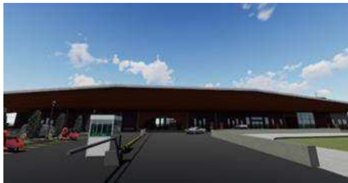
Figure 9. Front View of Ciamis Station
