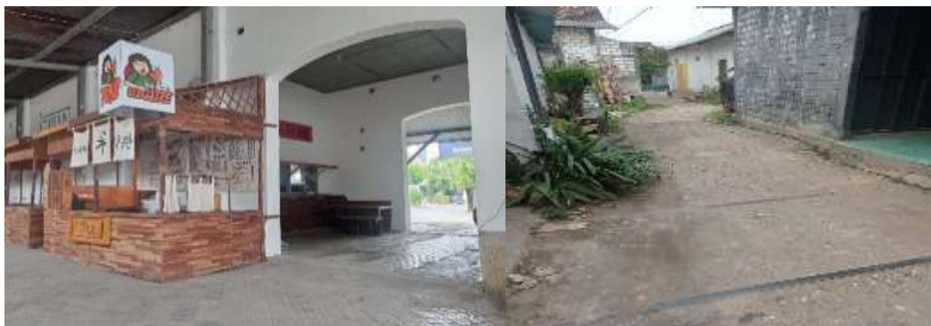
Figure 1. Existing Condition of Tuban Station
